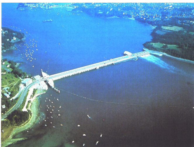
Figure 3: aerial photography of the La Rance plant
